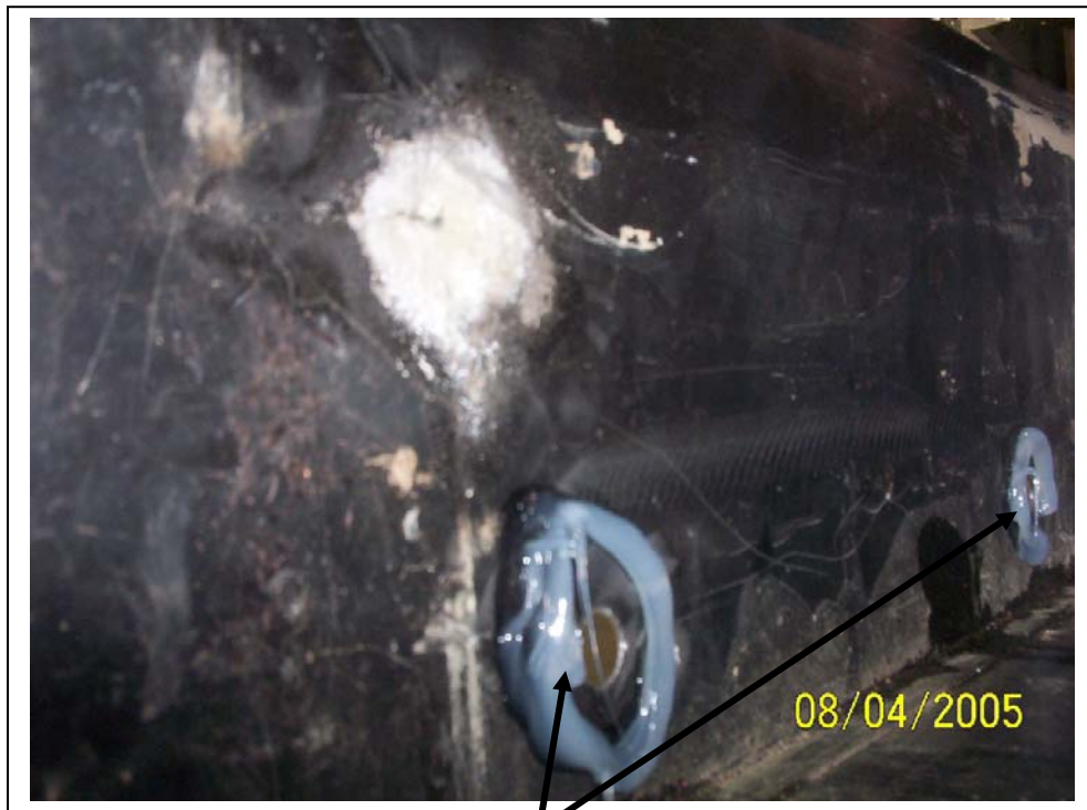
Silicone around drain tube holes then place drainpan in place. Ensure the drain pan holes are lined up with the box holes.
