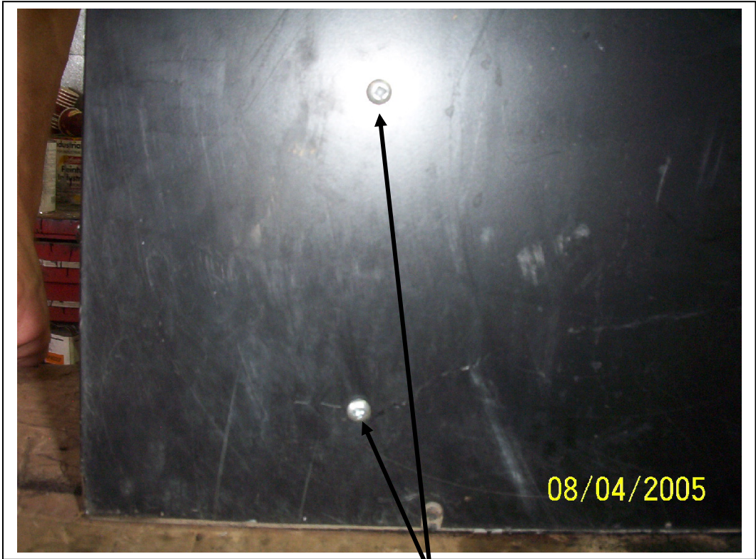
#8 self tapping screws used to mount the coil.
