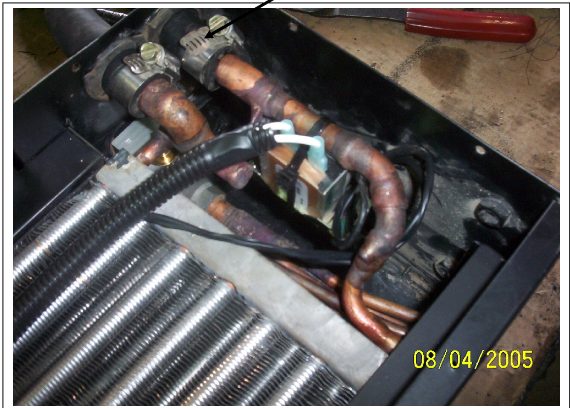
Re-use rubber 90° and gear clamps
