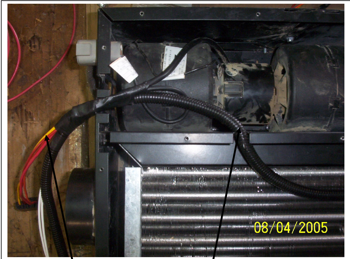
Electrical for power fans with 10" extensions.
